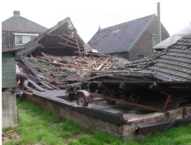
Fig. 5. Damage of a (old) barn due to the tornado in Muiden on 23 August 2004 (photo by R. Sluijter).
