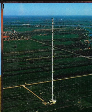
KNMI Meetmast Cabauw
