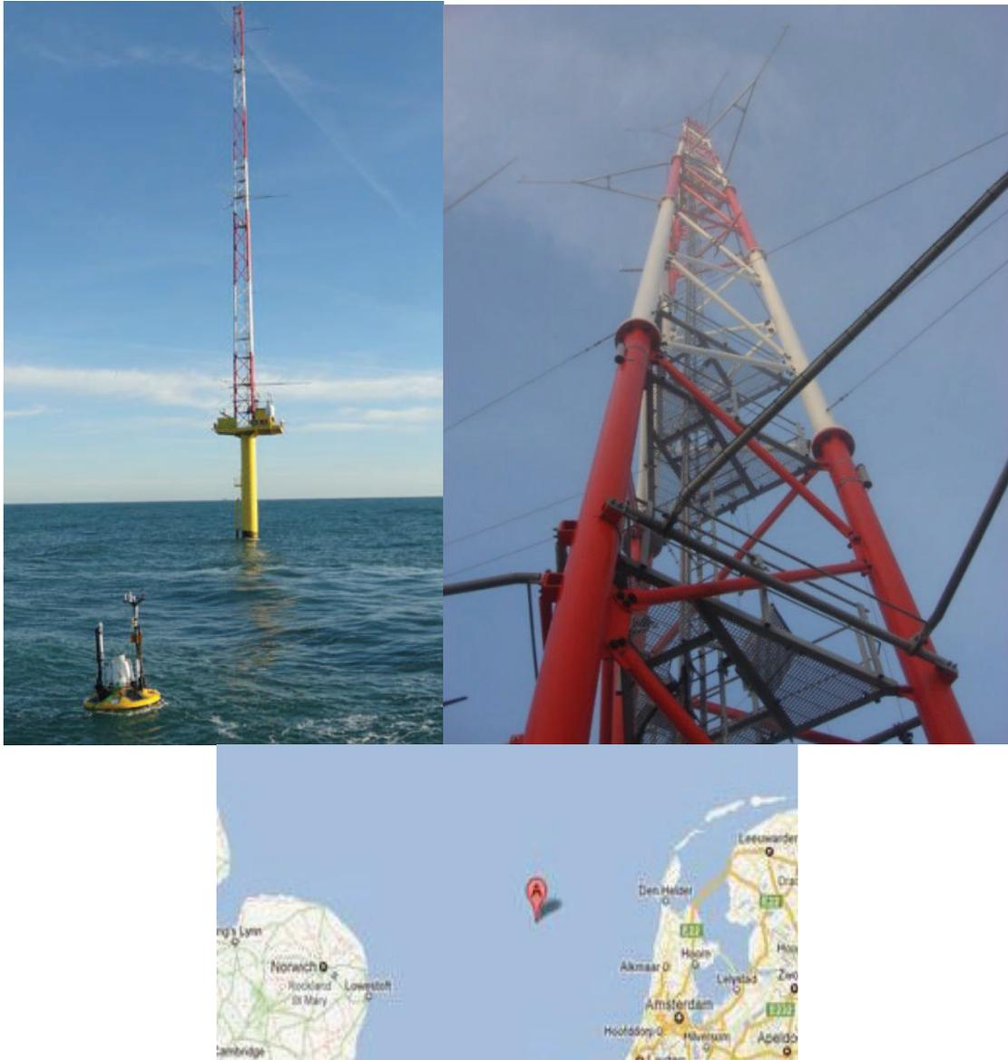
Figure 1: The top left panel shows Meteo Mast IJmuiden and the top right panel shows the mast construction and booms (source: BLIX Consultancy BV). The location of the mast is given in the panel below (source: ECN part of TNO).
