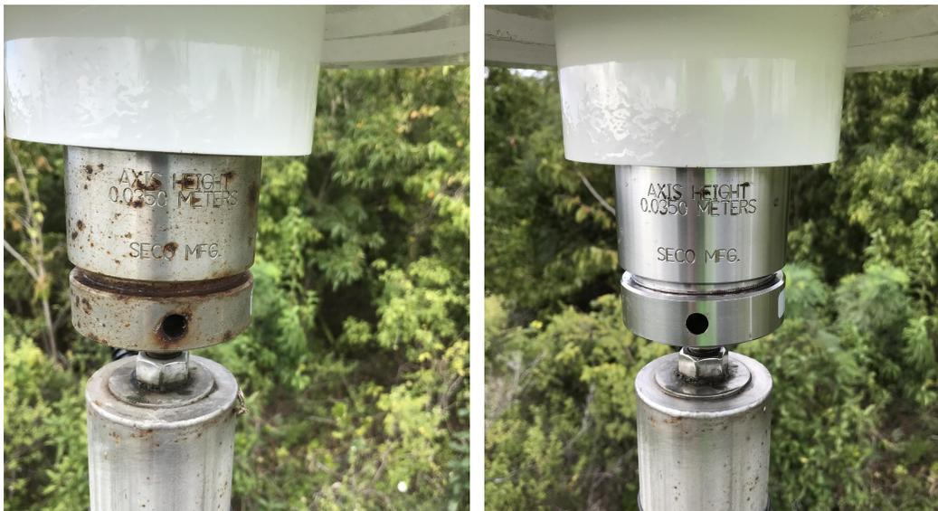
*Fig 2. Corroded stainless steel leveler after 1 year of exposure to the elements at White Hook (left). After maintenance the leveler looks as good as new (right).*
