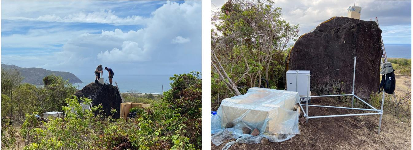
*Fig. 2: Drilling for the GNSS monument (left) and construction of the housing for the seismometer (right).*
