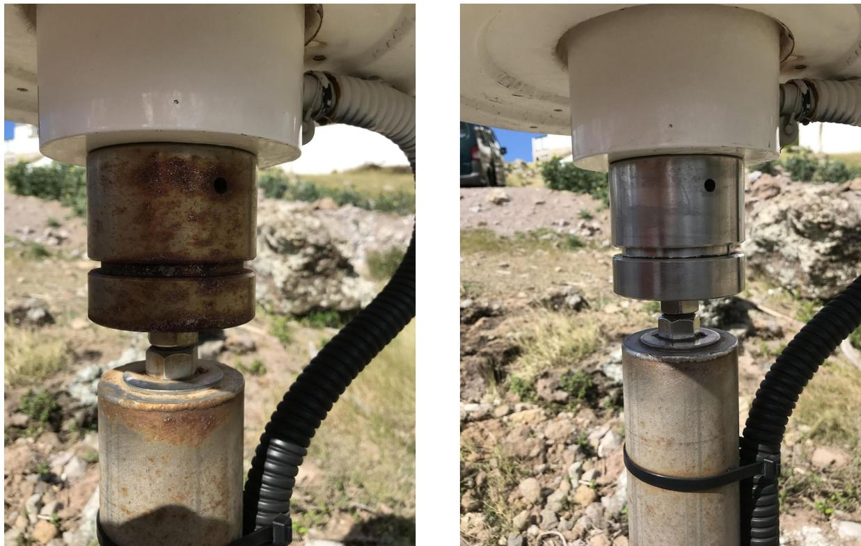
*Fig 2. Corroded stainless steel leveler after 1 year of exposure to the elements at St. John's (left). After maintenance the leveler looks almost new (right).*
