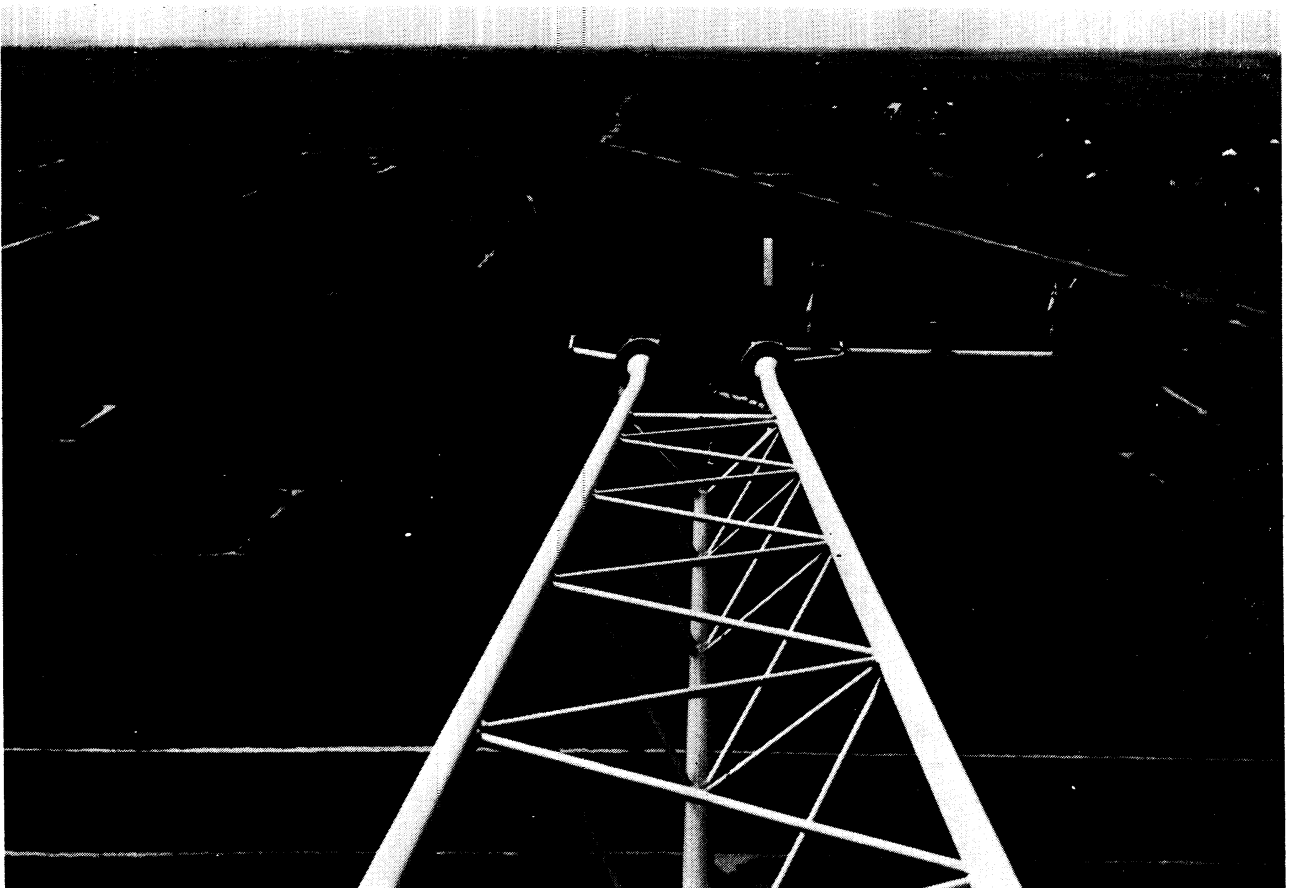
Fig. 4. View from 80 m mast level towards SW (direction Schoonhoven).
