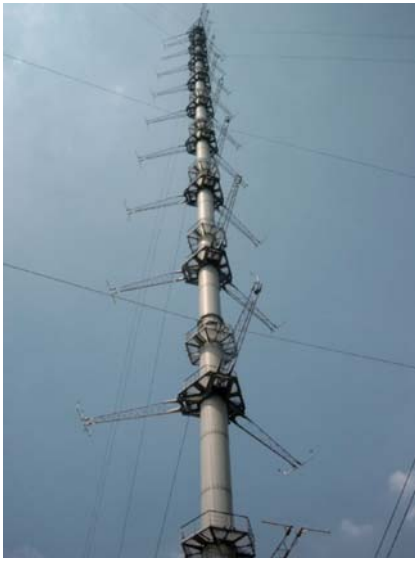
FIGURE B.3.1 213 m high Cabauw meteorological mast.
