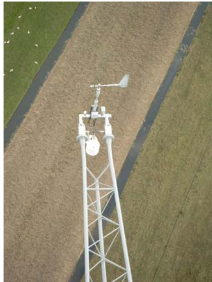
FIGURE B.3.4 Temperature and humidity sensor mounted on a boom in the Cabauw mast.
