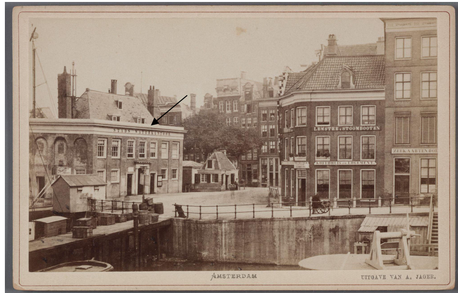
Figure 5: Location of the Amsterdam City Water Office at the Nieuwebrug/Zeerecht (1868–1878). The photo shows the Office housed in building 'Zeerecht' (as indicated by the black arrow). The Office was situated in front of the present Prins Hendrikkade 50, in former days Kampersteiger 10. Image obtained from the 'Amsterdam Gemeente Archief'.
