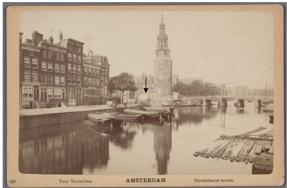
Figure 6: Location of the Amsterdam City Water Office at the Montelbaanstoren (1878–1963). The photo shows a view of the Montelbaanstoren with the Oude Schans canal. Right of the Montelbaanstoren the bridge over the Waaleilandsgracht is visible. The Stadswaterkantoor was situated in and around the first floor of the Montelbaanstoren (see arrow). Image obtained from the 'Amsterdam Gemeente Archief'.
