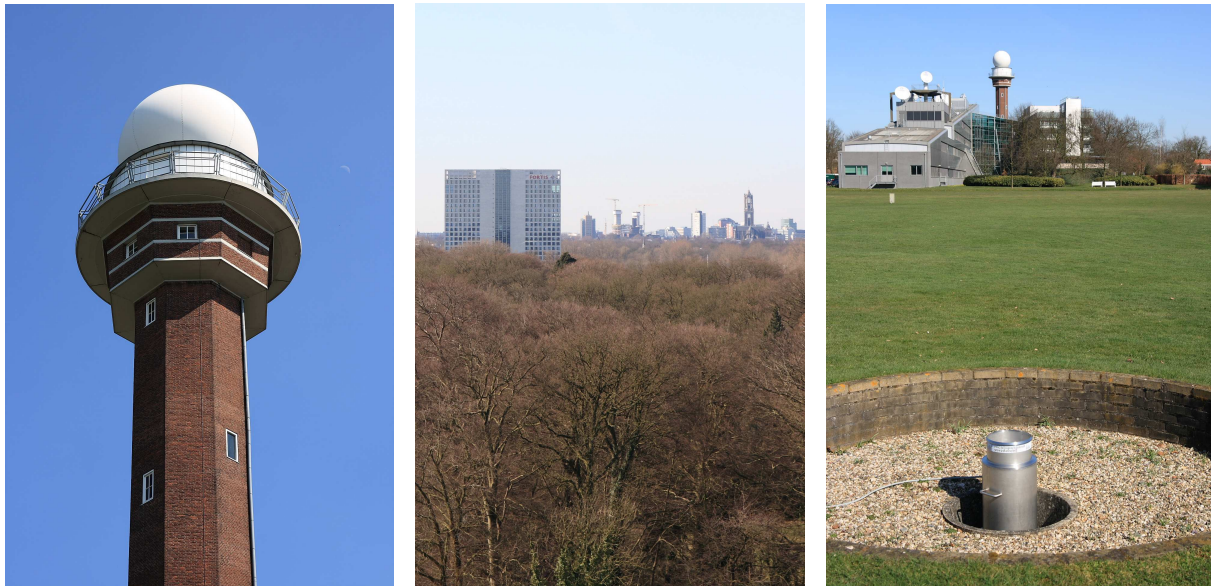
Figure 1.2: The radar tower in De Bilt, the Netherlands (left), view from the radar in De Bilt in the direction of a major building which partly blocks the lowest radar beam (middle), the best of two worlds (right): combine the rain gauge (in front) and the weather radar (background). The radome protects the antenna of the radar system.
