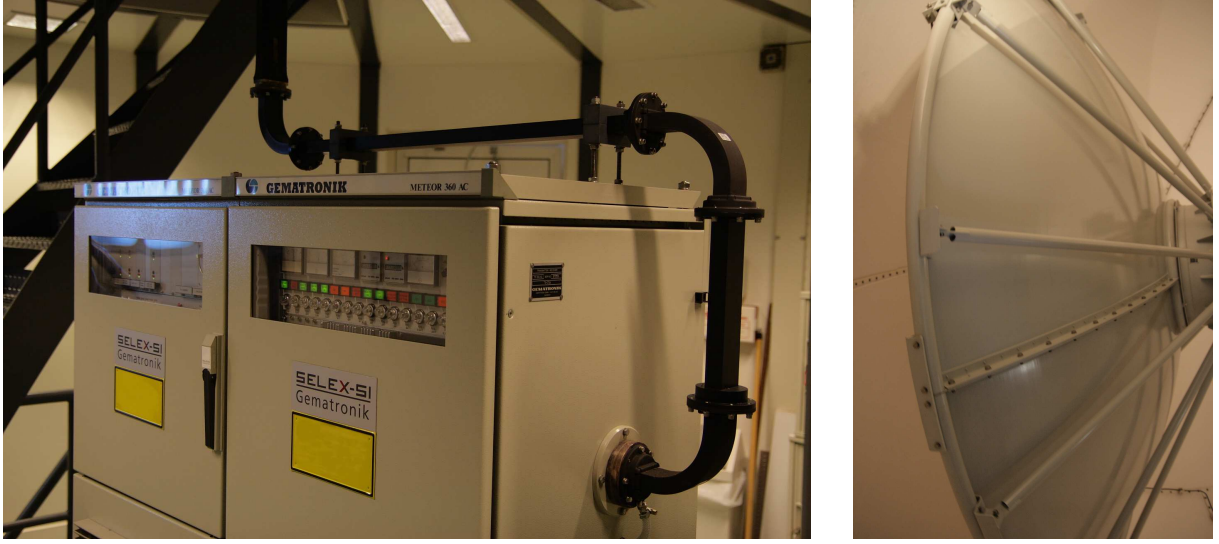
Figure 1.5: Transmitter cabinet, receiver cabinet and waveguide (left), and the circular parabolic reflector of the KNMI weather radar in De Bilt.
