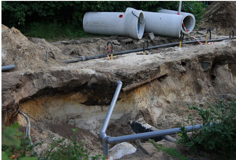
Figure 1.1: A sewer system under construction.
