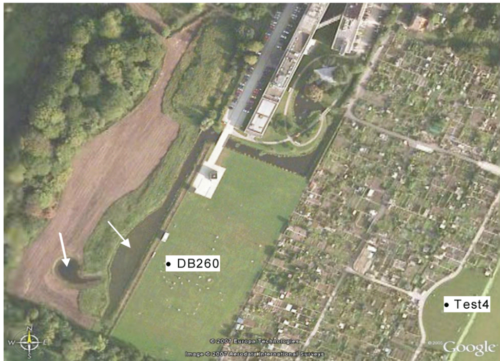
Figure 2.4: Aerial photo of the measurement field after the renovation of the wasteland area west of DB260 in September/October 2004. The arrows point to two new bodies of water.
