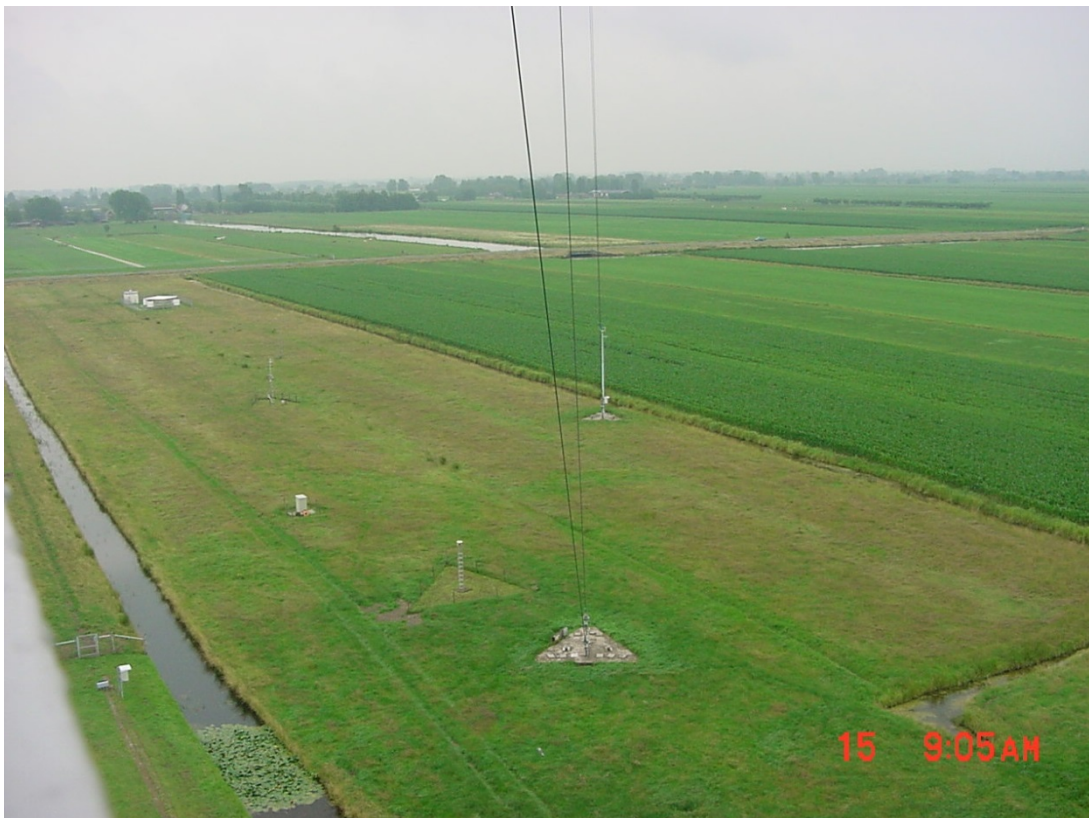
Figure 2 View from the main tower to the South. At the second guy-block close to the maize field is the 10 m tower of the automatic weather station. On the far end of the grass strip is the wind profiler/RASS system. The 5 m mast with turbulence equipment is positioned more or less in between these two configurations.
