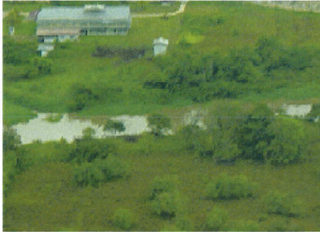
Figure 1.1: Paramaribo station and direct environment
