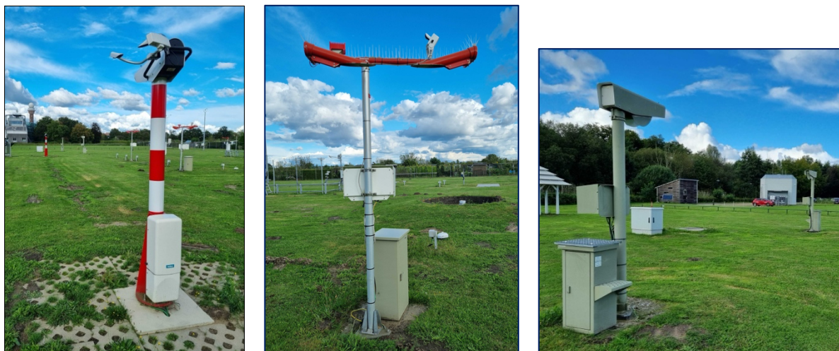
Figure 1: Visibility instruments. Left: Vaisala LT31 transmissometer Middle: Vaisala FD12P forward scatter present weather sensor Right: Vaisala Mitras transmissometer.
