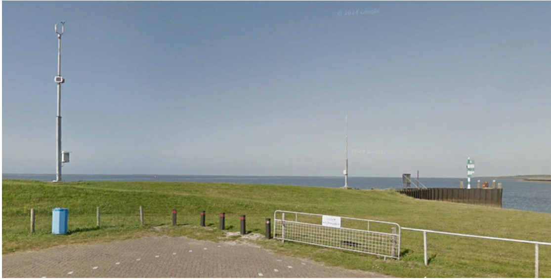
Figure F.16: Situational photo of the wind mast (left) at Lauwersoog (277).
